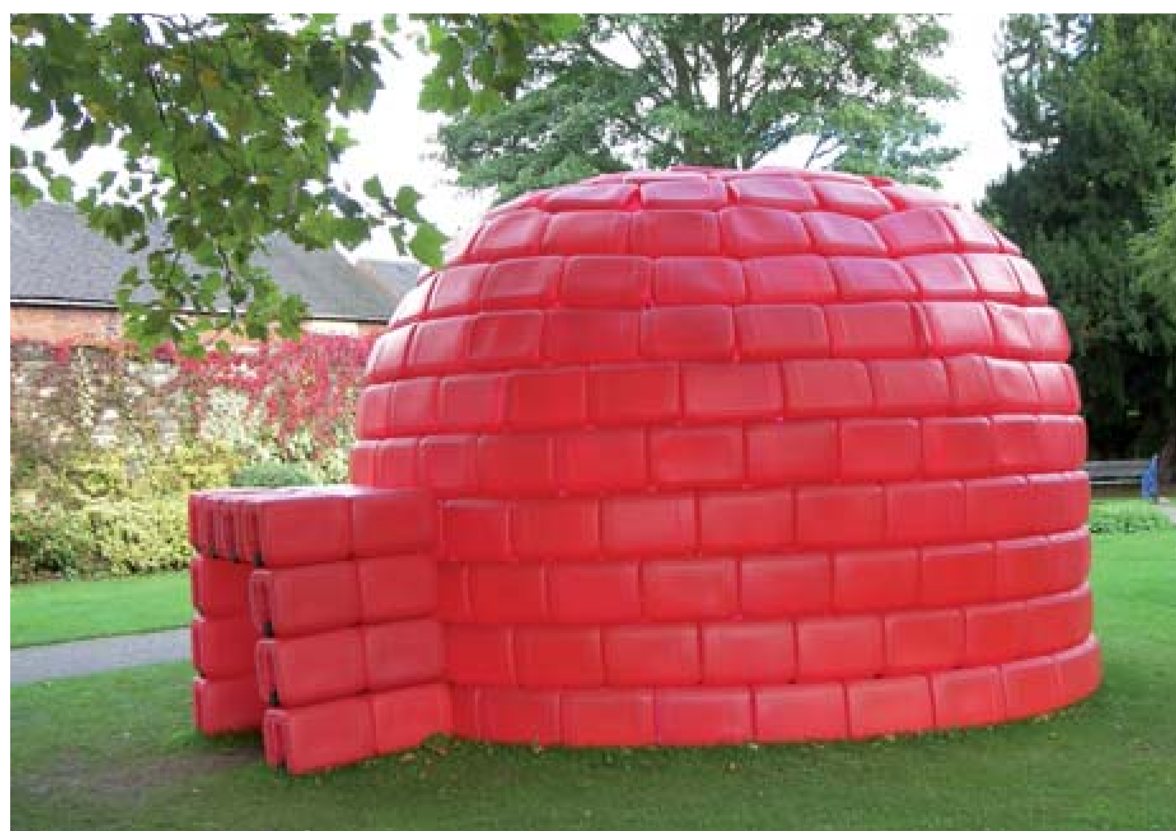
Bibigloo is made with 250 red PE recycled cans which are usually used as container for chemical products used in swimming pools.
